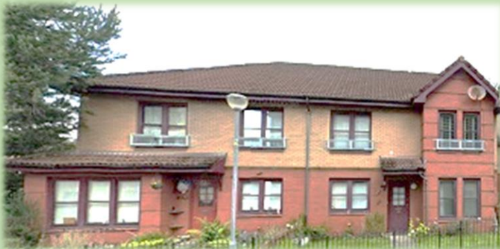
Before window replacement
