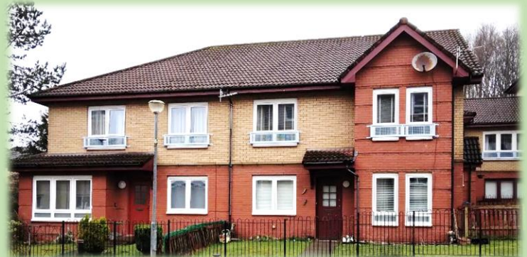
After window replacement
